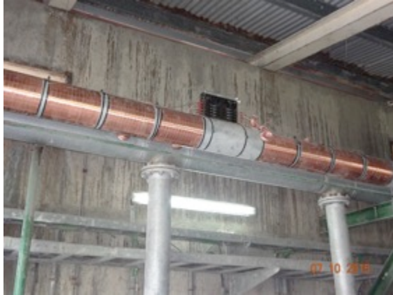
02 Vulcan S250 units on cooling tower water pipe
