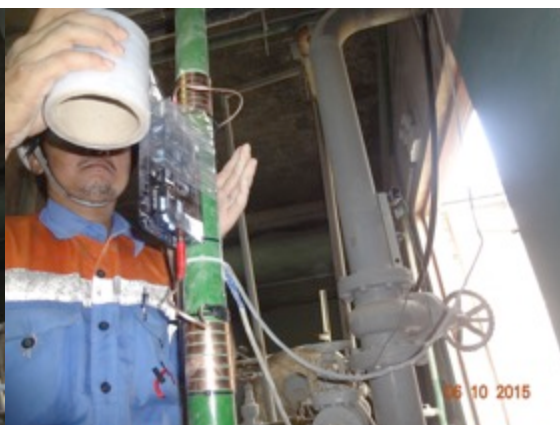
01 Vulcan 5000 on cooling tower of small grinder
