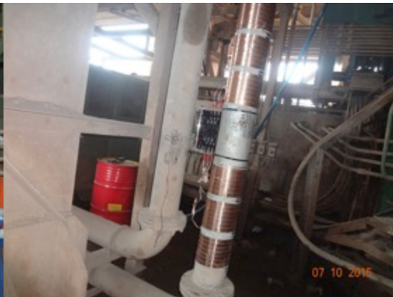
01 Vulcan S100 on cooling tower of big grinder
