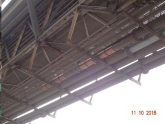
02 Vulcan S250 units on cooling tower water pipe
