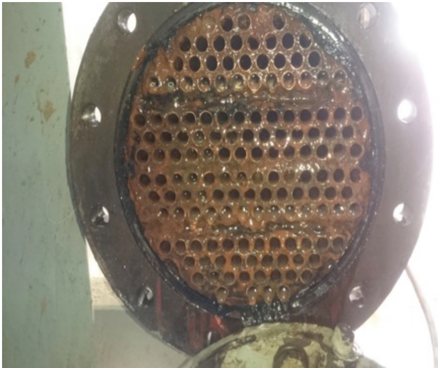
Heat exchanger before installation
