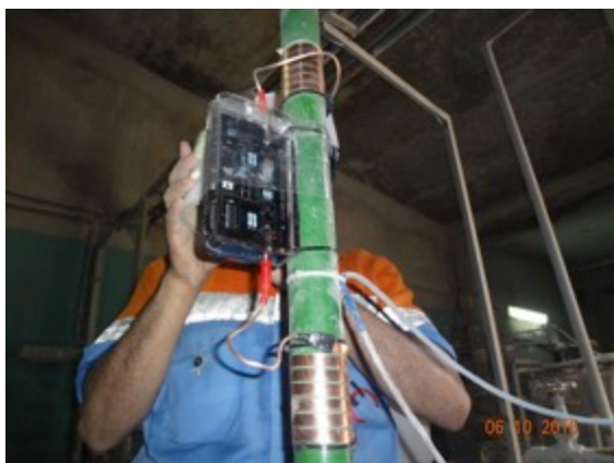
01 Vulcan 5000 on cooling tower of small grinder
